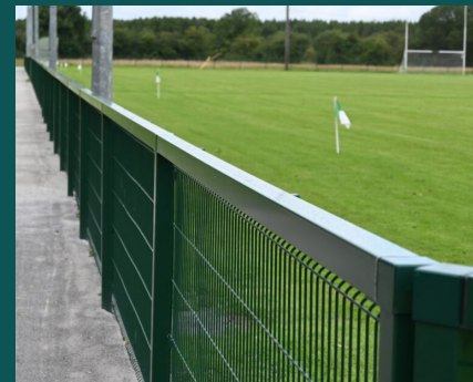
Ballyfore GAA - completed fence.
